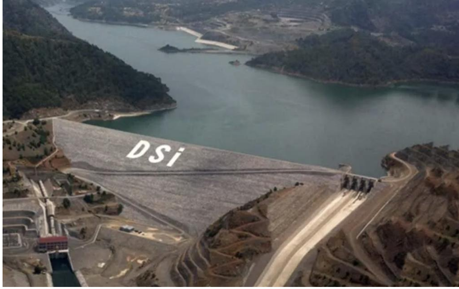
Figure 4: Akköprü Dam, Muğla [29].
